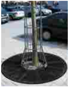
Tree protection in Hamburg / Germany
